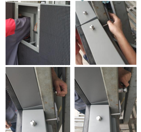
Step4: finish the other connect plate and bolt from front of the cabinet
